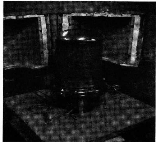
After installation of oxidation vessel
