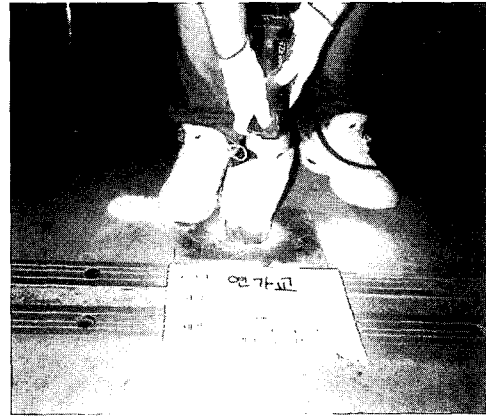
Fig. 2 Extraction of concrete samples
