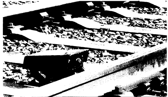
Fig. 5 Rail lubricator(side of rail)
