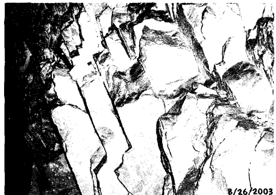
Fig. 3. Spalling of a pillar at Level D (405 ML) of Daesung mine
