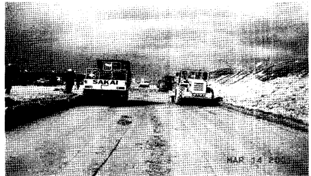
Fig. 9 Soil-cement compaction
