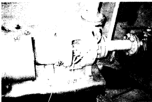
Fig. 3 Vibrational data acquisition set-up for the centrifugal pump
