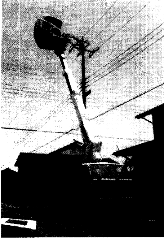
Fig. 1 Maintenance task of a 6-link electro-hydraulic manipulator
