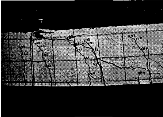
Fig. 11 Failure of slab No. 2.
