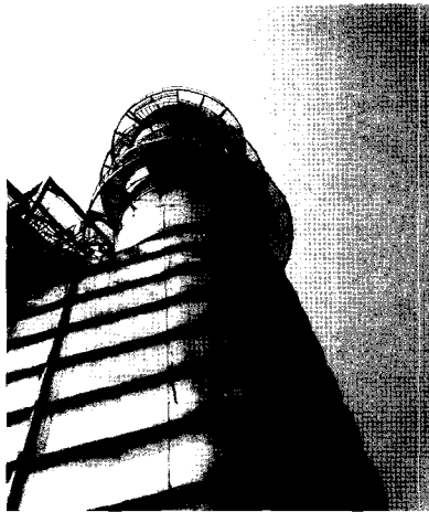
(d-2) Chimney of steam power generation
