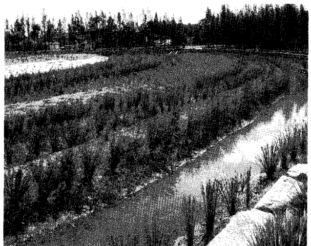
Fig. 5. Woodcroft park constructed wetland.
