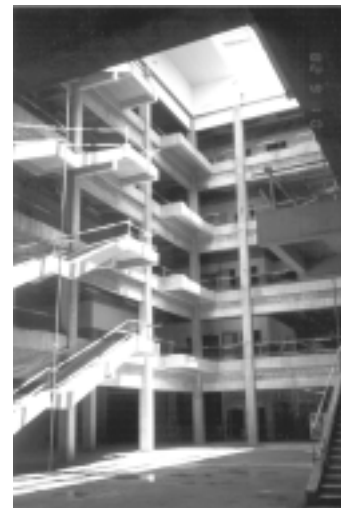
Fig. 12. Chang sha central Hospital
