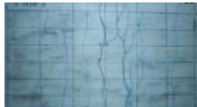
Fig. 8 crack type of sn08 specimen
