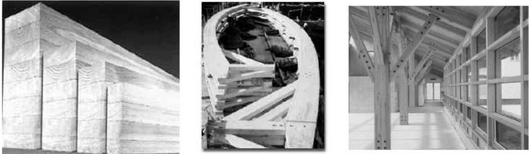
Figure 15. Application of tannin-based adhesive to cold-set glulam.
