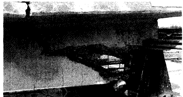
Fig. 10 Example of web shear failure (DT-2S-M-A)
