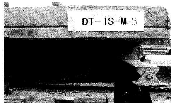
Fig. 11 Example of web shear failure(DT-1S-M-B)
