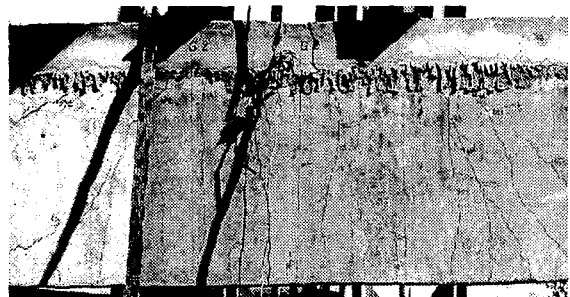
Fig. 12 Example of flexural crackings at failure stage (G-2)
