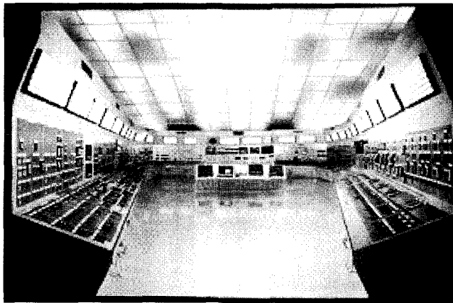
Fig. 2 Main control boards for seismic qualification
