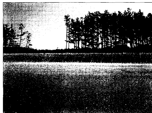
Figure 5. Seawall, Bagsajang, Tae'an
