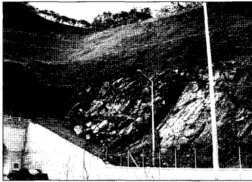
Fig. 5. Slope failure site of 2-A zone in S-2 area.
