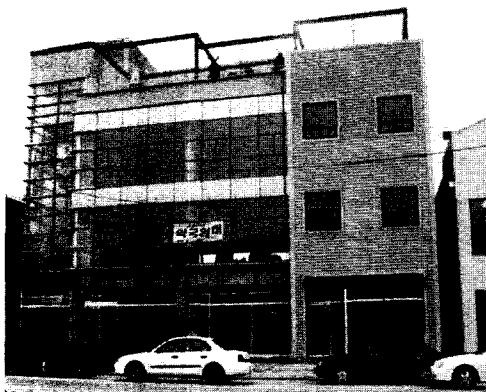
Fig. 6 Metal spray to steel wall Kangwondo, Gansung, 2002)
