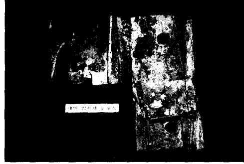
(b) No sprayed anticorrosive inside side panel
