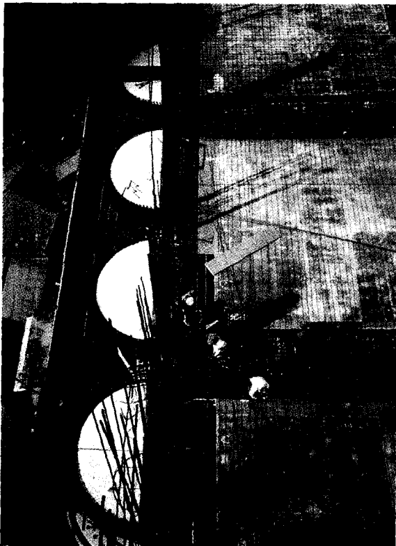
Fig. 8. Periphery frame tube and flat beam-slab system.
