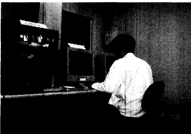
Figure 5. Computer systems for a production managing system, a plant operating system and a data base system located in the control room.
