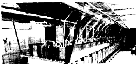
Fig. 10. A Single Phase Chain Link Converter – 16 Links
