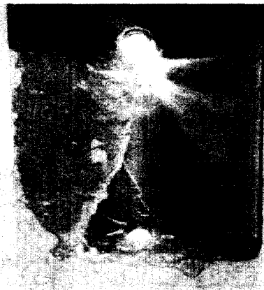
(b) Crack in bedding mortar
