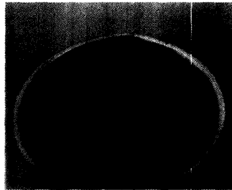
Fig. 1. Example of flange crack.
