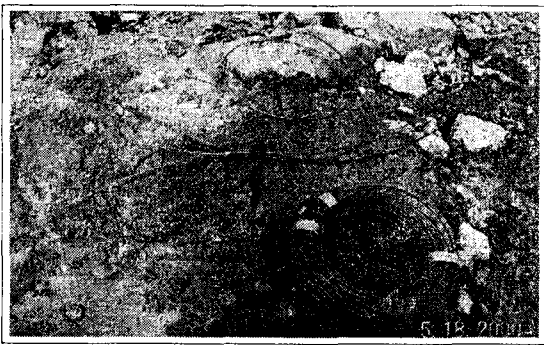
Fig. 7. Connection using the NONEL
