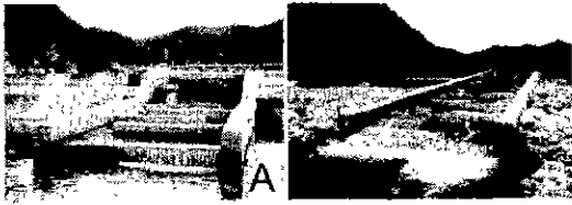
Fig. 5. Improved baffled fishway at Bukpyung weir(A : before improvement, B : improved)
