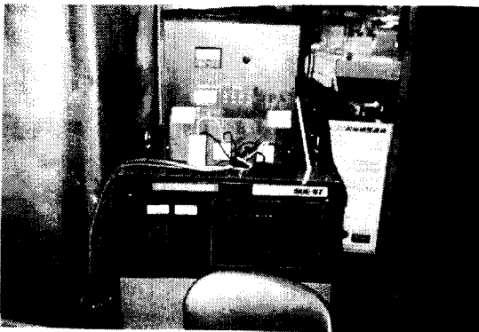
Fig. 4 Power Supply Unit
