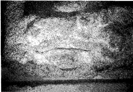
Fig. 6. Right 3 face of the fore-room; dark brown weathered surface, crack development and high relief surface by weathering.
