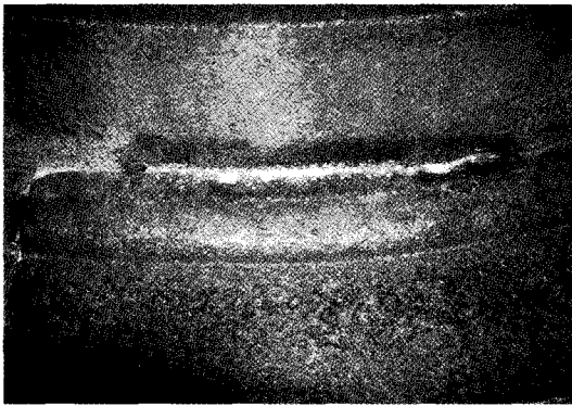
Fig. 9. Rear of the seat; black color due to influences of cement weathering in the contact.
