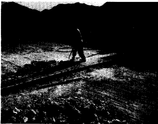
2. Expansion Joint 제거
