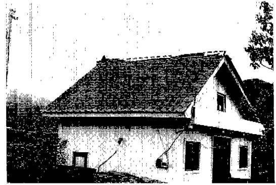
Fig. 2-7. Falling of the roof tiles on the house at Yongjang-ri.
