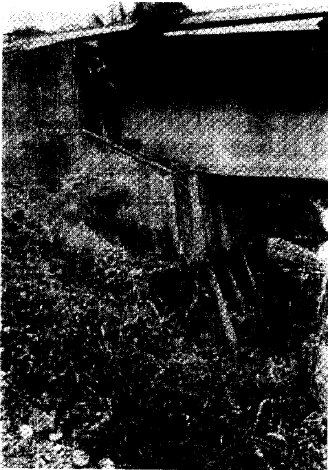
Fig. 3 Abutment slumping and rotation failure Rio Banano bridge, 1990 Costa Rica earthquake
