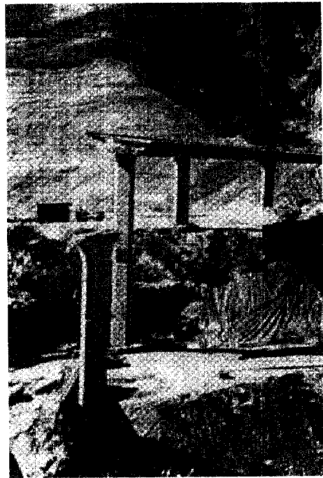
Fig. 1 Span collapse, 1971 San Fernando earthquake
