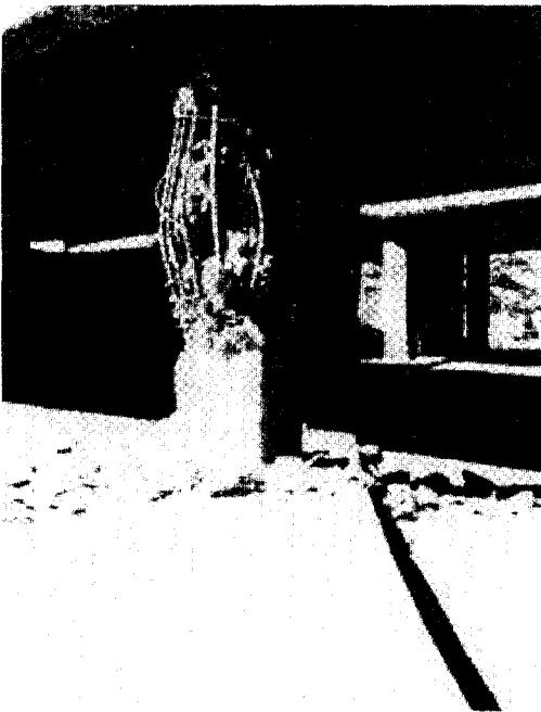
Fig. 6 Shear failure outside plastic hinge region, 1971 San Fernando earthquake
