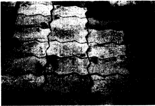
Fig. 3. U type wooden block set up exterior site.
