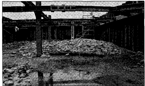
Photo 2. Before excavation. Ancient bridge foundation.
