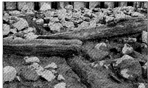
Photo 3. Wooden bridge foundation. Softwood used for base structure.
