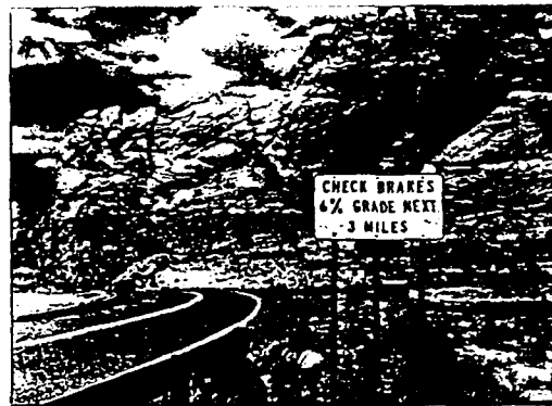
그림16. A brake check area created at the top of a grade in Arizona.
