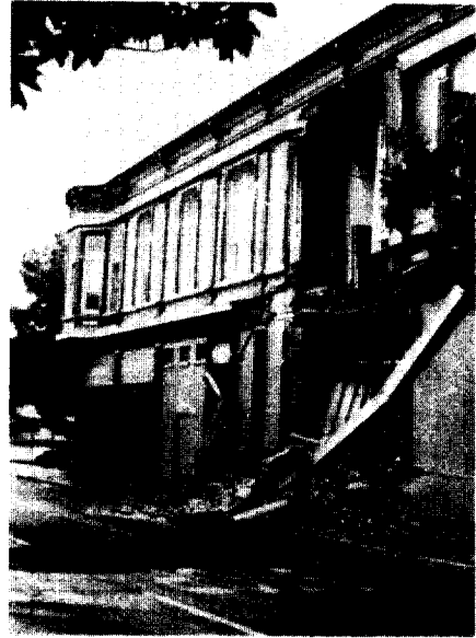
Photo.7 Out-of-plane failure of URM all at center of building due to excessive diaphragm flexibility (Santa Cruz, Loma Prieta Earthquake)
