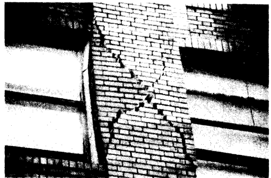
Photo.4 In-plane shear failure of URM pier (Oakland, Loma Prieta Earthquake)
