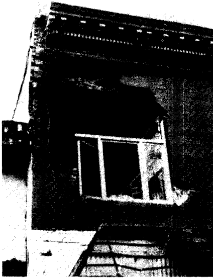
Photo.12 Combined out-of-plane/ pounding failure (Santa Cruz, Loma Prieta Earthquake)
