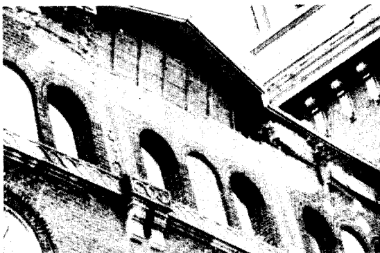
Photo. 10 Failure due to combined out-of-plane failure of parapet and inadequacy of collar joint in multiwythes URM wall(Quebec City, Saguenay Earthquake)
