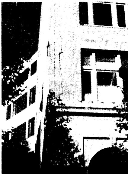
Photo.13 Diaphragm-induced corner damage to URM pier(Oakland, Loma Prieta Earthquake)
