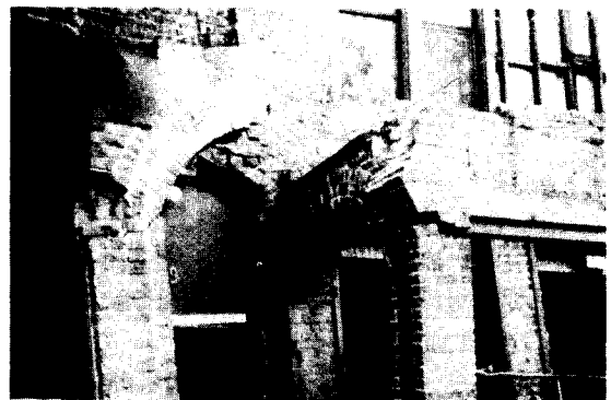
Photo.5 Flexural failure of slender URM column (Los Gatos, Loma Prieta Earthquake)
