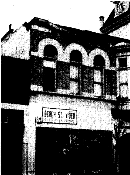
Photo.8 Parapet failure of 100 front street building (Watsonville, Loma Prieta Earthquake)
