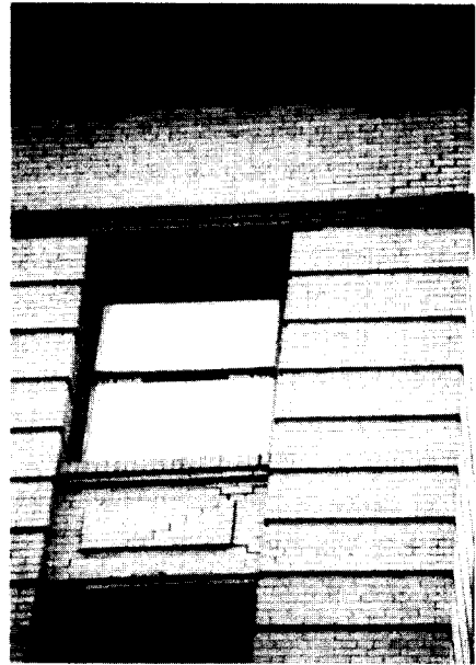
Photo.3 In-plane shear failure of URM spandrel beam (San Francisco, Loma Prieta Earthquake)
