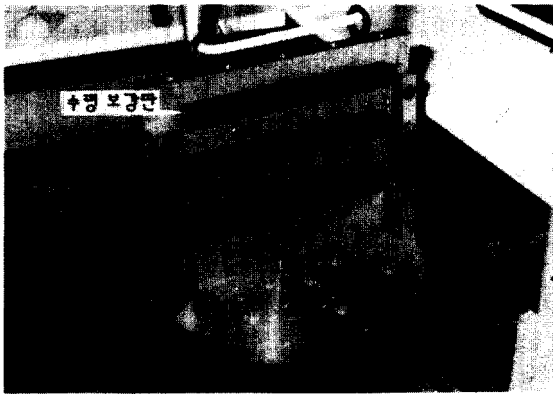
Fig 10. Horizontal Gussets
