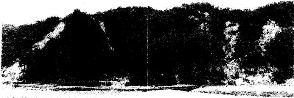
Photo 1. Landslides in Hamyang site.
