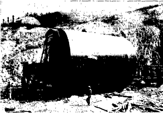
〈사진-1〉 Needle Beam Type Circular Steel Sliding Form
