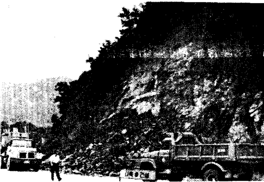
Fig. 4. Treatment by the rock slope greenification
