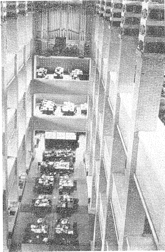
〈사진 13〉 FRANK LLOYD WRIGHT, Larkin administration Building, Buffalo, 1904. Nave with surrounding galleries.
