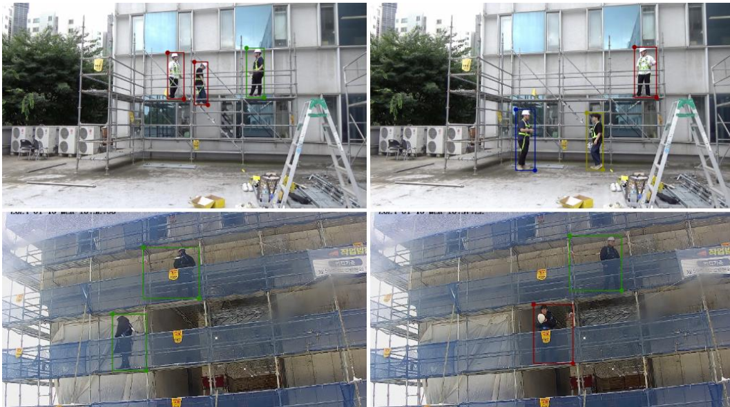
Figure 2. Visualization of safety assessment testing images with bounding box annotations. Green boxes represent height-safe, red boxes represents heigh-unsafe, yellow boxes represent ground-unsafe, and blue boxes represents ground-safe. Some workers were annotated as occluded for being covered by other objects without proper vision to the workers.
