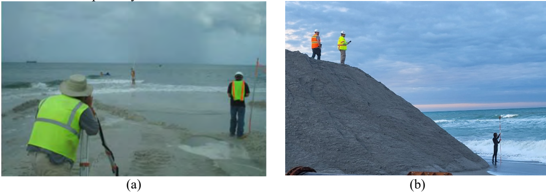
Figure 2: Topographic survey collection of the beach berm and slope in the surf zone [2].
