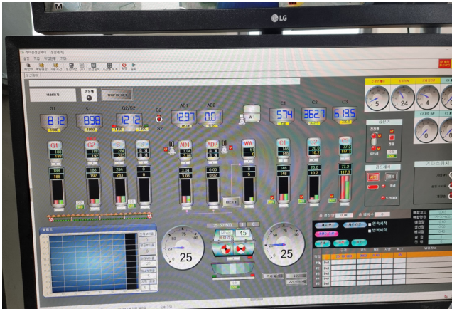
Figure 1. Concrete batcher plant road control
