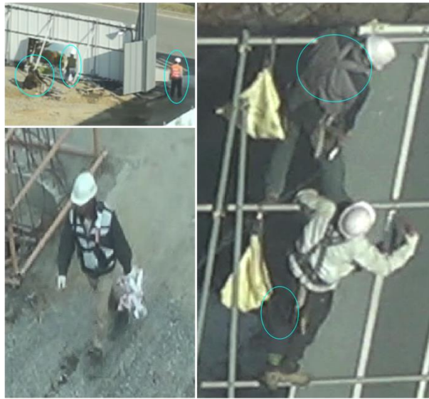
Figure 1. Example of collected YUD-COSA images. The varying object sizes, color similarity, and object thickness create difficulties in workers and PPE recognition for far-field safety monitoring. Limited optimization in loss functions can lead to unreliable monitoring.
