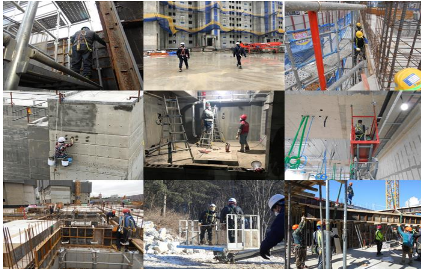
Figure 2. Images collected at construction sites
