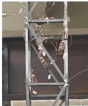
Figure 5. A segment of the Structure Lab Structure
