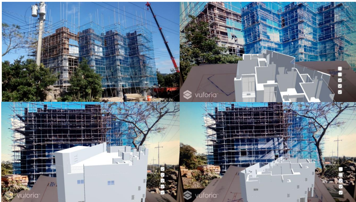
Figure 6. Views of the real building under construction and the AR model
