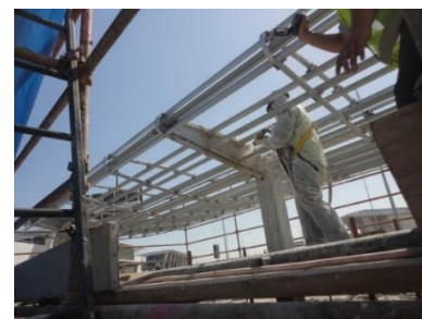
iii. Skylight Area
