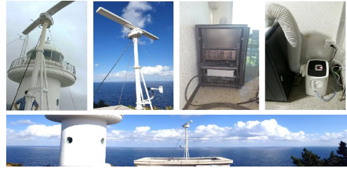
Fig. 2 Installation and facilities of x-band marine radar for wave monitoring on Dodong light house
